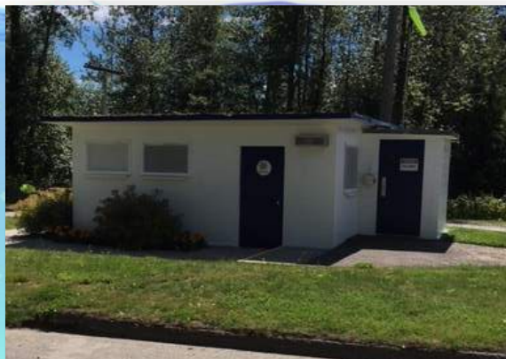
In town Chlorinator, located just before the bridge.
