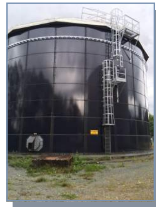
New steel reservoir from 2014
