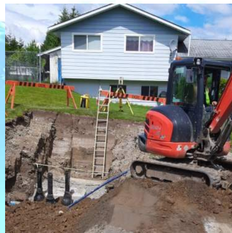
Water Main Repair
