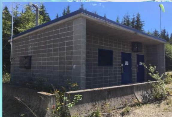
Cable Car Chlorinator, located on highway 37 across from Cable Care entrance.
